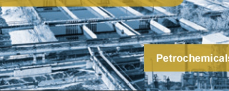
Purification and recycling plants
